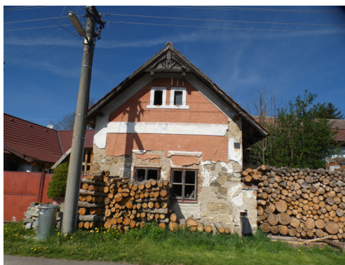
Fig. 1.: Front view of the house in Horosedly, author: J. Rolínková (Source: photo author)
