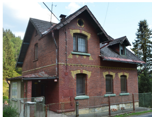
Fig. 9.: Bublava house No. 481 – double-colored solid burnt brickwork with yellow bricks used for window arches, cornice, ornament under the windowsill, and window lining of a circle window in the upper part of the gable. [Source: Dominika Výšková (photograph), 2023].
