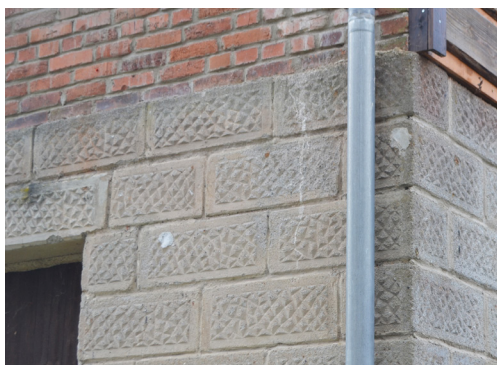
Fig. 7.: Bublava house No. E75 – basement masonry made of prefabricated concrete blocks with rustication. [Source: Dominika Výšková (photograph), 2024].
