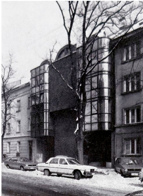
Fig. 7.: CHB in Vodovodna St, Zagreb, 1983; Author: Radovan Tajder (Source: [13])
