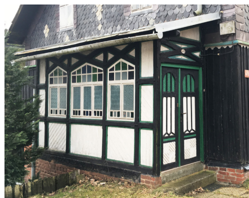
Fig. 8.: Bublava house No. 475 – half-timbered construction of entrance hall called Schneehaus with a window made of multicolored glass plates. [Source: Dominika Výšková (photograph), 2024].
