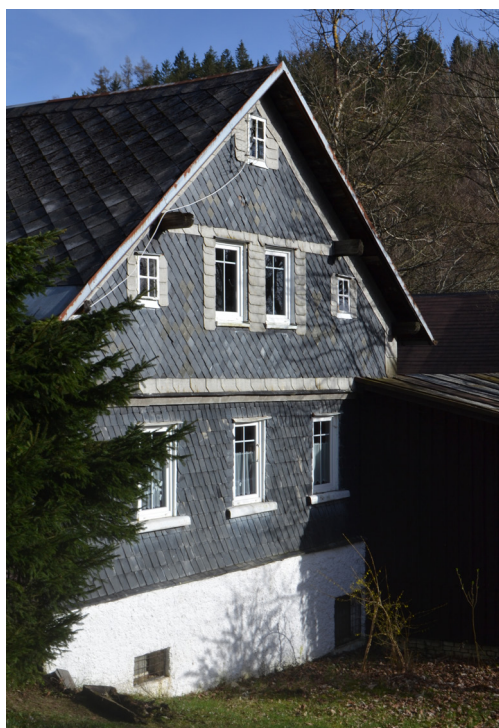
Fig. 12.: Bublava house No. 34 – a rare example of façade finishing made of slate templates in the Kraslice microregion. [Source: Dominika Výšková (photograph), 2024].
