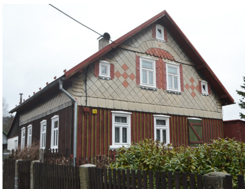
Fig. 6.: Bublava house No. E142 – artistically valuable cladding of eternite templates. [Source: Dominika Výšková (photograph), 2024].
