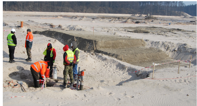
Fig. 4: Trial construction site and coring of cylinders for E-modulus test
